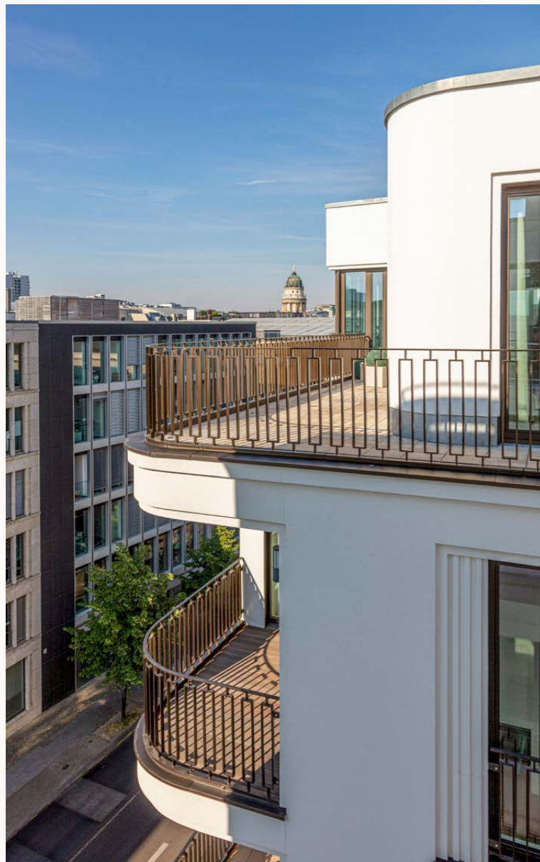
Detailansicht der Penthouse-Terrassen / Detailed view of the penthouse terraces
